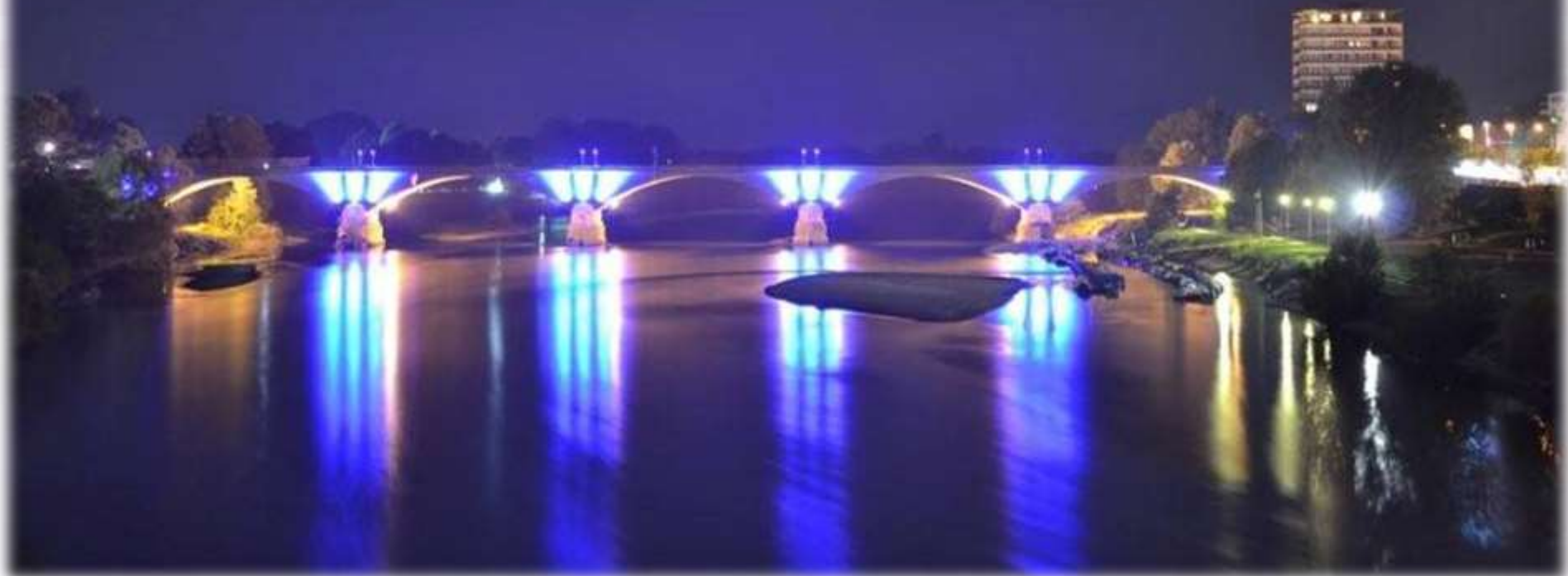
Photo: view of the modern bridge of Pavia
